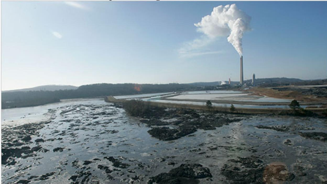
*Three hundred acres were covered with toxic sludge in late December when a wall of a coal ash holding pond near Kingston in East Tennessee gave way.*
