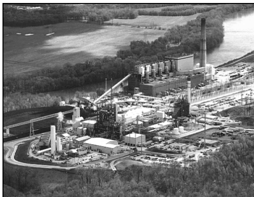
Wabash River IGCC Project West Terre Haute, Indiana
