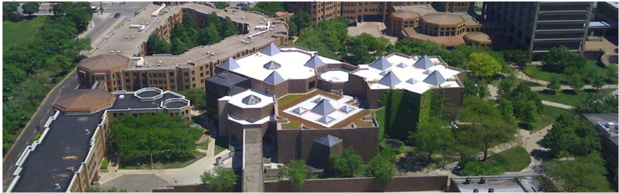
Figure 14: Green Roof on Art & Architecture Building
