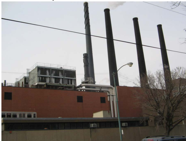
Figure 8: Power Plant – West Campus
